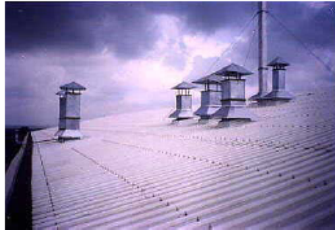
PVC roofing material
